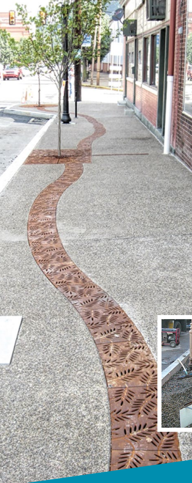
Installation of trench drain, tree grates, and downspout disconnect
