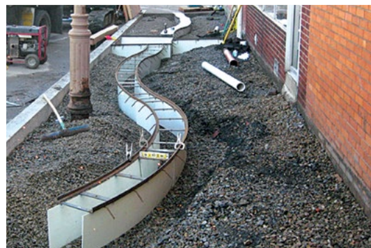
Installation of trench drain, tree grates, and downspout disconnect
